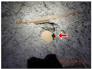
(2) There is less than the current required amount of insulation in the attic ceiling area for our climate zone. Current construction standards for our climate zone specifies R49 as the attic insulation value. You may consider adding additional insulation in the attic in the future for additional energy efficiency. Your current installed value is approximately: R19 - R25
