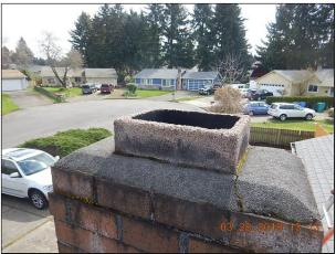
(2) There is significant deterioration of the chimney crown mortar and the brick mortar. Deteriorated chimney crown mortar may allow moisture penetration and further crack / deteriorate the crown and the mortar between bricks is crumbling and soft. I recommend repair by a mason.
