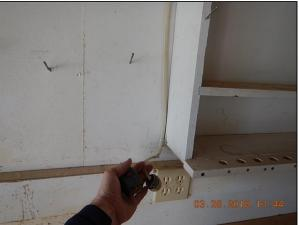
(5) There is some electrical cabling in the crawlspace / attic which appears to be abandoned. There was no voltage at the cabling / outlets. I do not know if there is potential for this to be energized. I recommend having it removed as there is no real necessity for it. Note: any outlets in crawlspaces should be GFI protected
