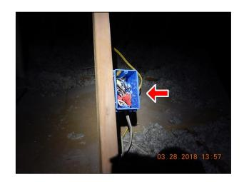
(4) There is non-professional type of wiring in some areas of the garage that I recommend an electrician review and correct for safety. The wiring is not properly installed / protected.
