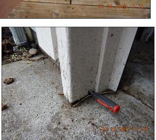
(6) I recommend not fastening fencing to the home's siding. This can trap water behind the board(s) and damage the siding / structure. I recommend a fence post at least 1 inch away from siding.
