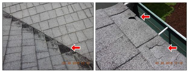
(2) The roof appears to be at or near the end of its life expectancy. The roof should be further evaluated by a licensed roofer to determine useful life remaining and I recommend budgeting for replacing the roof covering. I estimate the roof covering will need to be replaced within the next 3 years, but repairs are necessary now.
