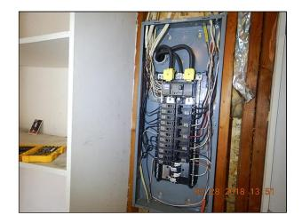
(2) There are multiple defects noted in the main electrical panel or auxiliary panel. Issues noted, but are not limited to: breakers are not clearly labeled for quick location in an emergency (safety item), white neutral wires used as hot and not relabeled multiple neutral wires under one terminal, wire jackets not stripped back to within 1 inch after entering panel. I recommend review and repair as necessary by a licensed electrician.
