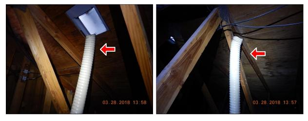
(3) The bathroom exhaust duct is made of flexible vinyl or foil. I recommend replacement by an insulated smooth walled metal or semi-rigid metal exhaust pipe to prevent potential condensation and damage to the ceiling.
