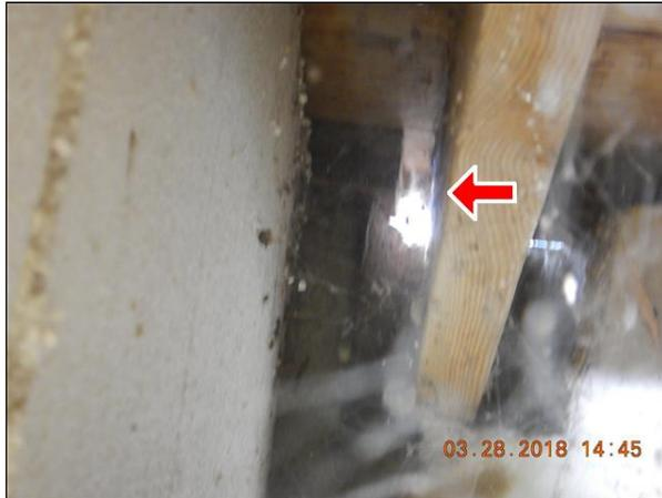
(4) The construction debris, insulation laying on ground, etc needs removing from the crawlspace under home. This could contribute to potential pest intrusion.
