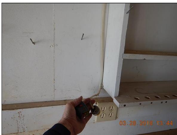
👉 (5) There is some electrical cabling in the crawlspace / attic which appears to be abandoned. There was no voltage at the cabling / outlets. I do not know if there is potential for this to be energized. I recommend having it removed as there is no real necessity for it. Note: any outlets in crawlspaces should be GFI protected
