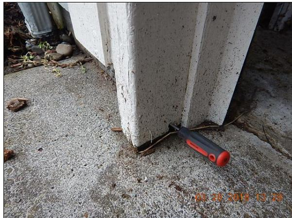
🔧 (6) I recommend not fastening fencing to the home's siding. This can trap water behind the board(s) and damage the siding / structure. I recommend a fence post at least 1 inch away from siding.
