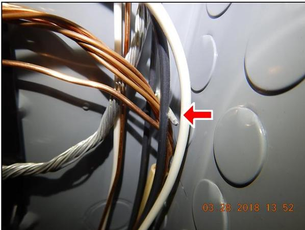
(4) I recommend covering the exposed wires at the bottom of the panel board to prevent accidental damage / contact.
