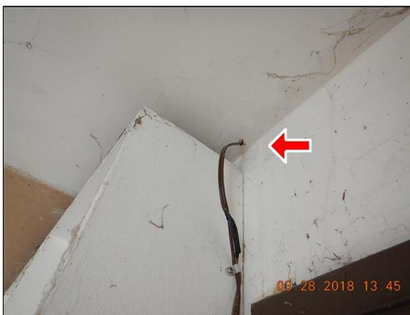
🔌 (2) One or more electrical outlets around the home did not have voltage at the outlet. Recommend repair by a licensed electrician. Areas noted: garage North / outside wall (multiple)
