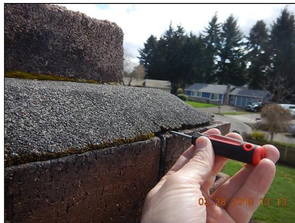
🔍 (3) The rubber boot of is a plumbing vents is cracked and / or gapping away from the vent pipe which could allow leaking either now or in the future. Monitor and replace as necessary. Noted: one plumbing boot is just starting to crack
