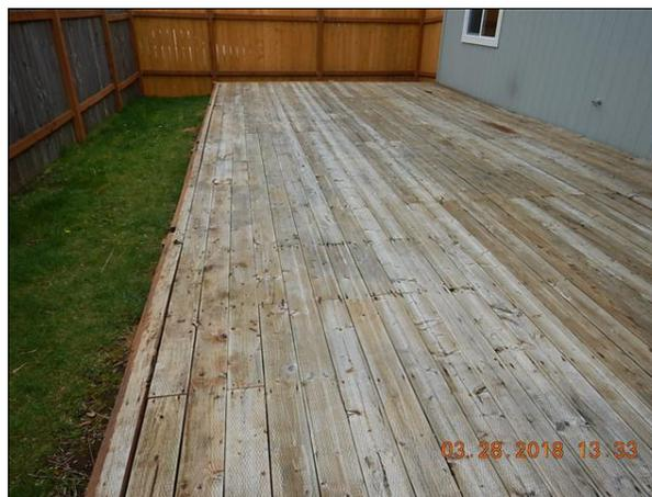
(2) The deck structure has been modified. The old railing has been cut off. The rim board / outside beam area is not supported but is bolted to the columns. Deck structure is in contact with the soil. Minor wood rot noted in deck. One loose board at rear of deck needs replaced. There are some things that will require repair going forward, but it is functional at present. Monitor and repair as necessary.
