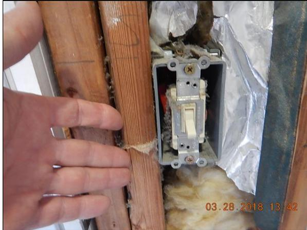
(3) There are one or more broken electrical receptacle or light switch cover plates. I recommend repair. Areas noted: garage
