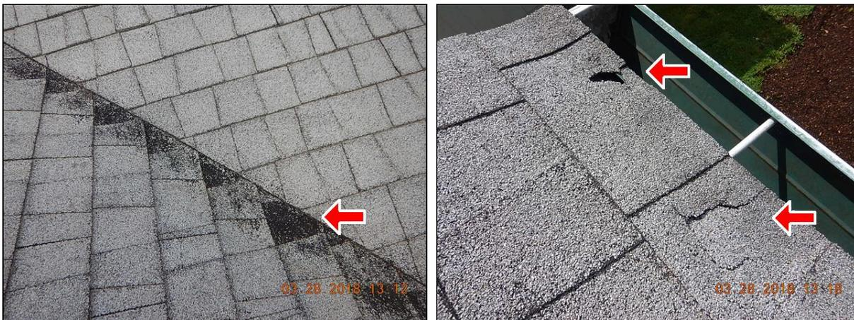
💰 (2) The roof appears to be at or near the end of its life expectancy. The roof should be further evaluated by a licensed roofer to determine useful life remaining and I recommend budgeting for replacing the roof covering. I estimate the roof covering will need to be replaced within the next 3 years, but repairs are necessary now.
