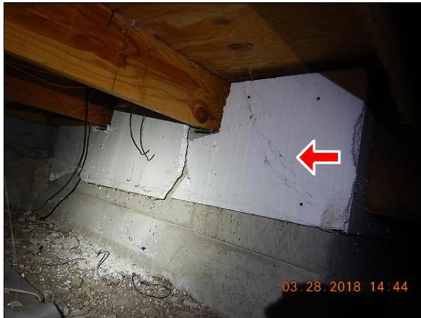
(3) There are some visible gaps into the crawlspace at the chimney area that can be sealed / foamed to prevent pest entry.
