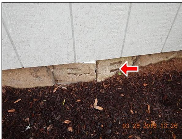
(2) The crawlspace vents are at or below the ground level in some locations. Recommend repair of landscaping to always keep crawlspace vents above grade to prevent moisture intrusion.
