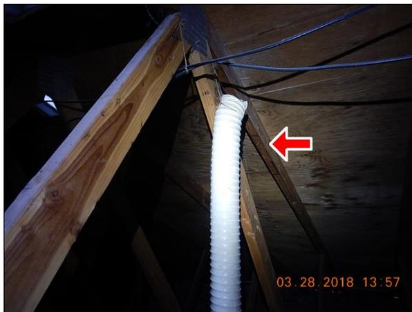
(3) The bathroom exhaust duct is made of flexible vinyl or foil. I recommend replacement by an insulated smooth walled metal or semi-rigid metal exhaust pipe to prevent potential condensation and damage to the ceiling.
