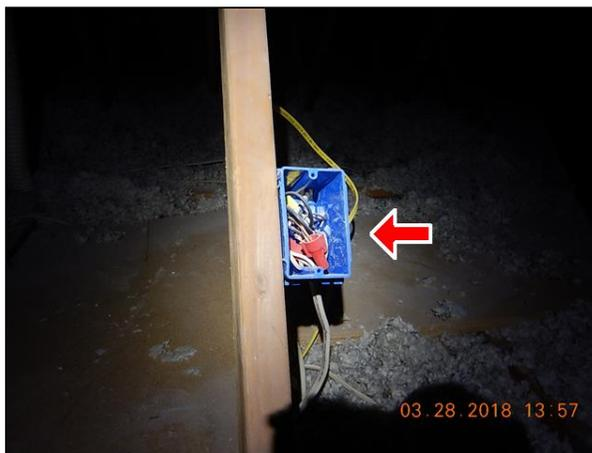
⚠ (4) There is non-professional type of wiring in some areas of the garage that I recommend an electrician review and correct for safety. The wiring is not properly installed / protected.
