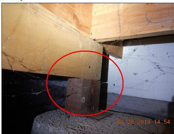
(2) There is a non-typical beam configuration in one area where the beam has been shimmed with a 2x4. I see no issue as a result, and it seems to be performing OK as-is.
